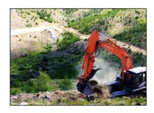
Rye Creek: Reduce streambank erosion to improve the fishery and reduce excessive sediment delivery to the Bitterroot River. Enhanced a riparian area using bioengineered bank stabilization, effectively rebuilding streambanks using willows and woody debris, and halting unnatural bank erosion. Rye Creek is one of the largest sediment contributors to the Bitterroot River; this project prevents excessive sediment from reaching the Bitterroot River.
