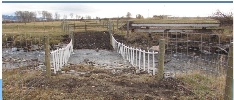
Guided cattle crossing at North Burnt Fork Creek concentrates passage to eliminate streamside damage associated with unmanaged, open access.
